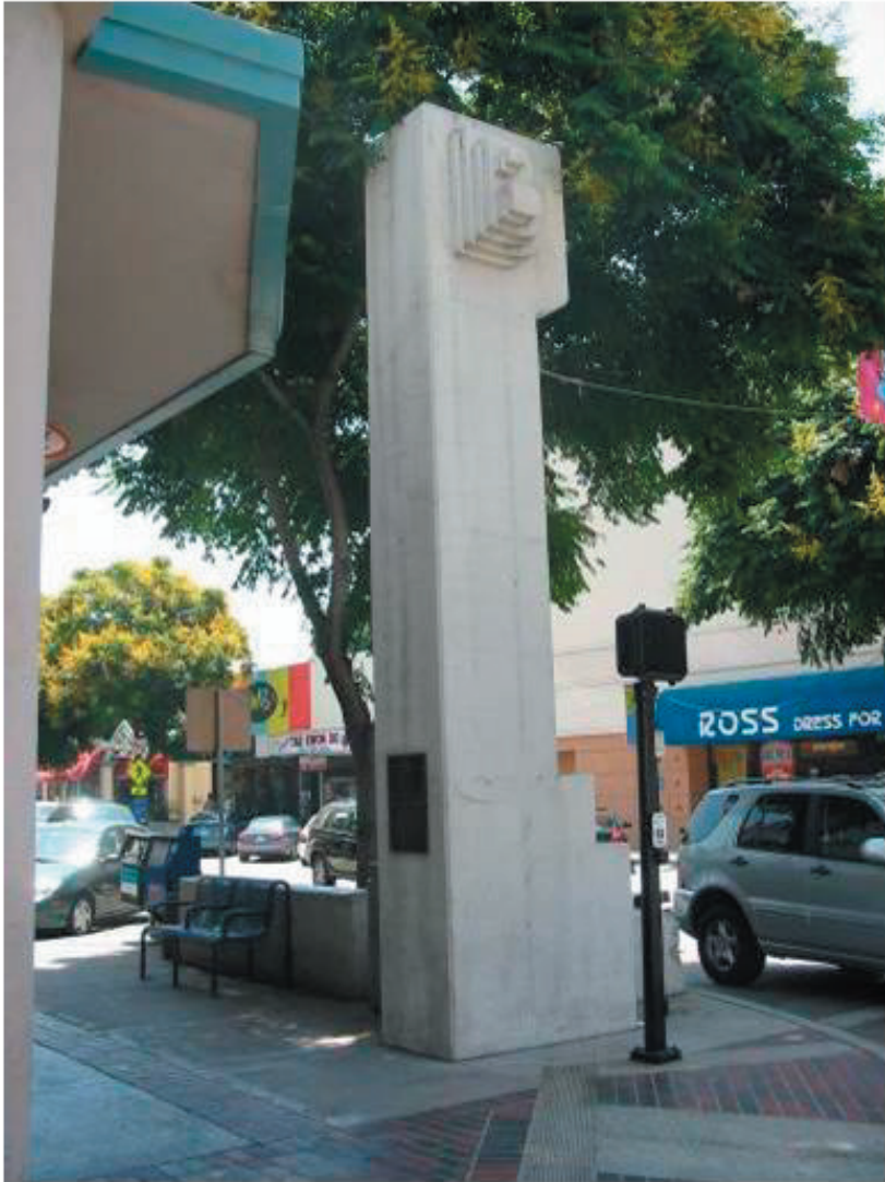
Existing Concrete 'B' Monument
